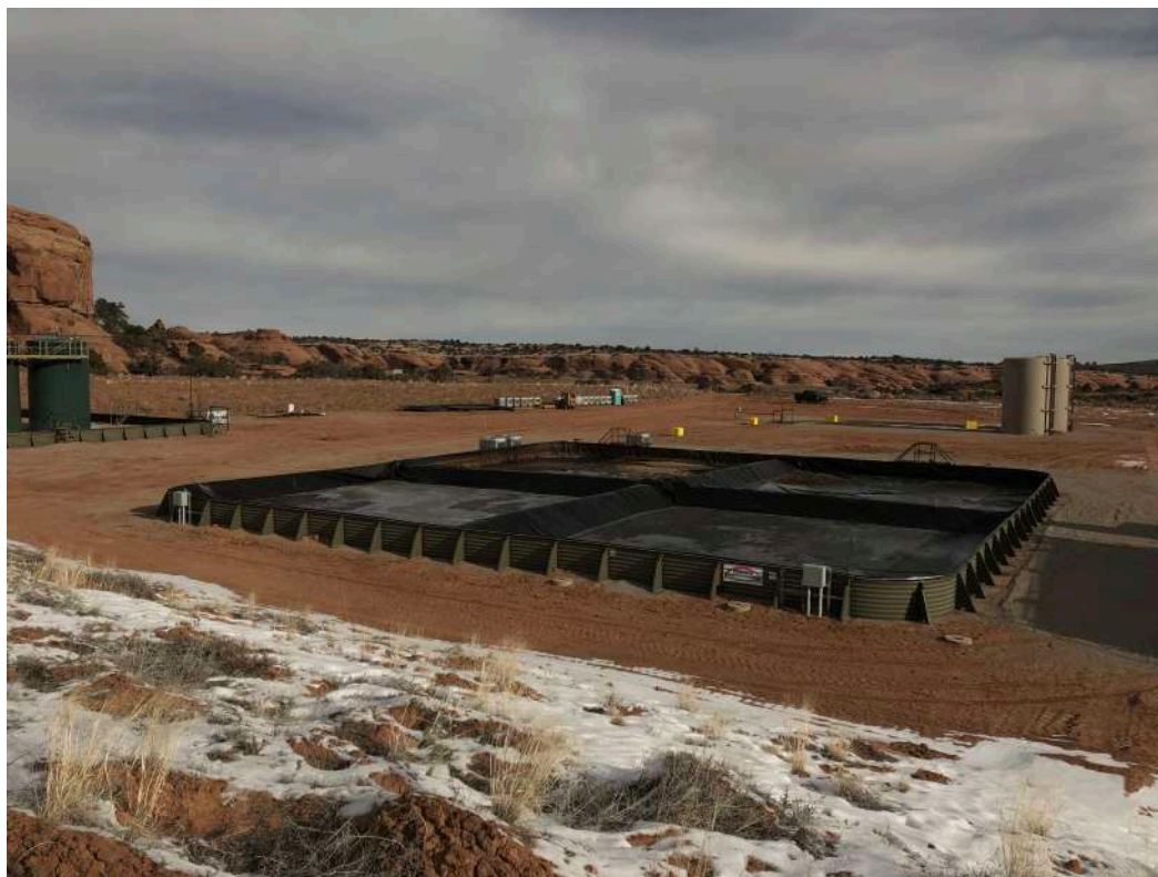
Figure 1: First stage of cleaning up of the bunded area after completion of evaporation testing.
